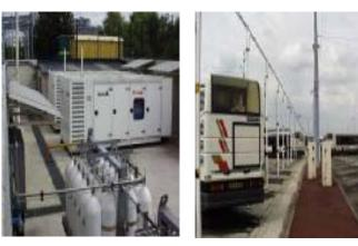
Large slow-fill system (Typically 15-30 buses or refuse trucks overnight) Size: 400-1,600 kg/hr This is unlikely to be used for Sprinters as there is far too much gas. Unless Sprinters share filling with other vehicles such as Econics
