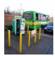
Medium slow-fill system Size: 10-20 kg/hr Sprinter: 117 – 234 km/hr 20 kg/hr for 8 hours would give 160kg = 1872 km = 187 km each for 10 Sprinters
